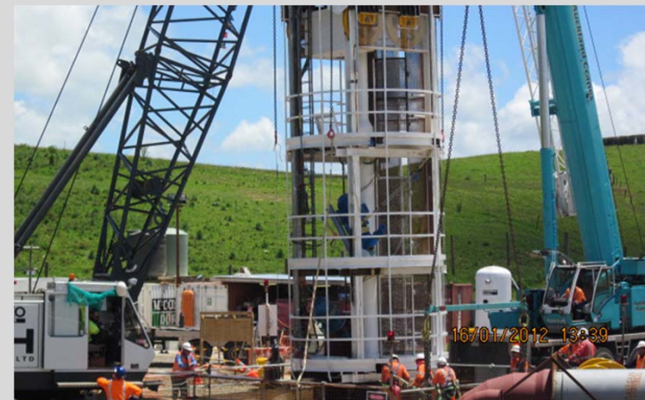
Huntly East Mine ventilation shaft ($30M)
