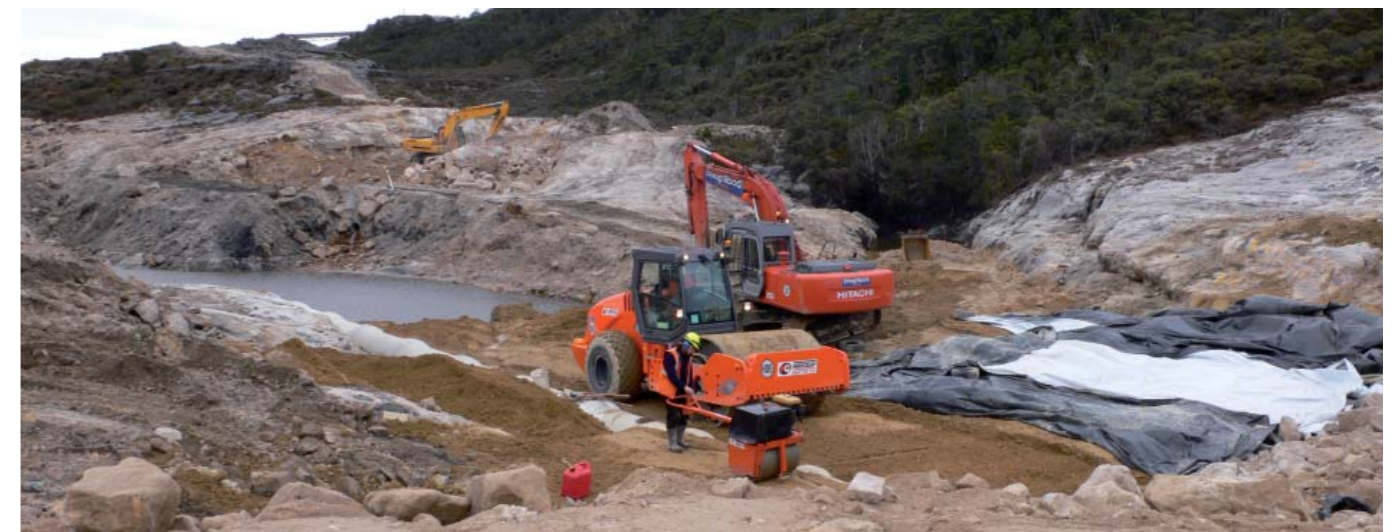
Dam construction works underway at Stockton.
