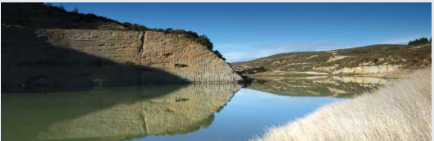
Mining highwall plunges into the lake (mid 2004)
