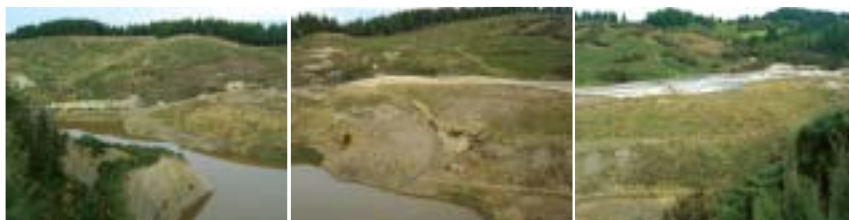
View from top of highwall over lake, waste rock hill and hillside behind (May 2005)
