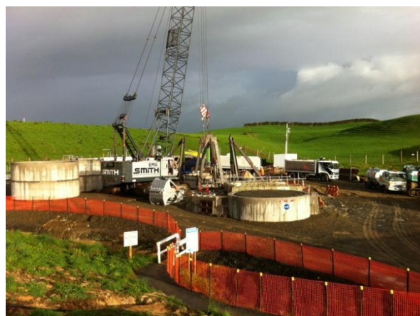
Huntly North Shaft – Commencing Caisson Support Construction
