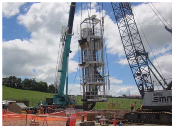
Huntly North Ventilation Shaft
